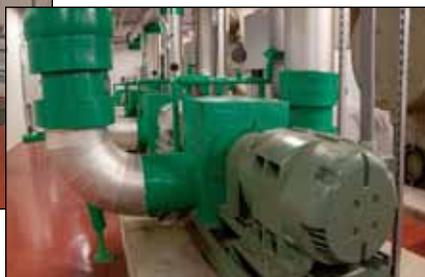
The satellite chiller plant is connected to the central energy plant and serves as a "stage" plant to provide chilled water for air conditioning needs on campus. It is connected through a 1 ½ mile underground piping loop. Equipped with three 1500 ton, 200 hp Trane centrifugal chillers (plus one as backup), the plant also comes with six 200 hp Taco TA pumps, multi-purpose valves, suction diffusers, a CA expansion tank and ABB VFD units to control the pumps.
